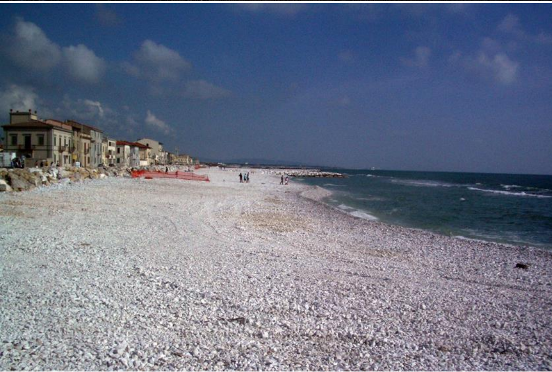
Detached breakwater lowering at -0.5 m Gravel beach creation
